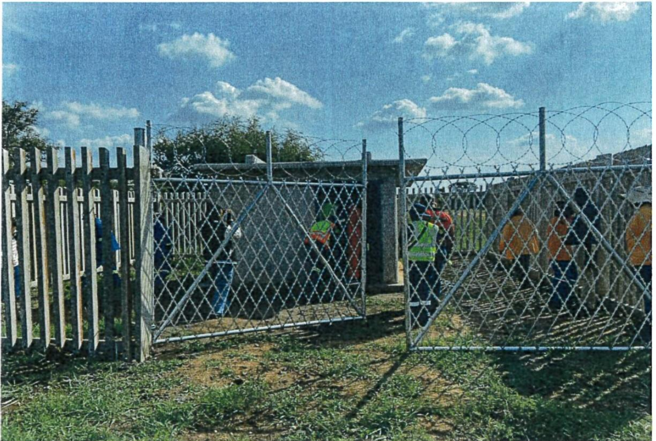
DAVID KATNAGEL PUMP STATION UNDER CONSTRUCTION
