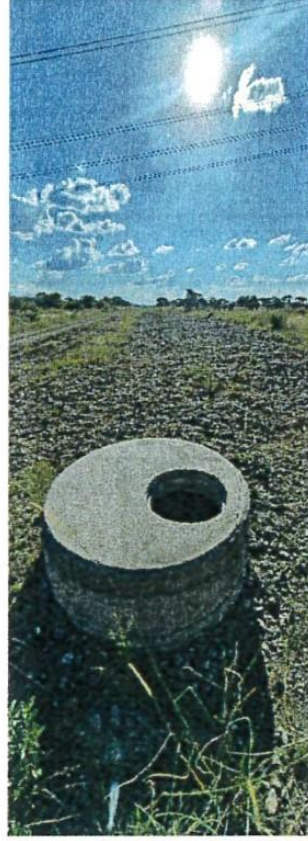
Completed Manhole Chambers and Rehabilitation
