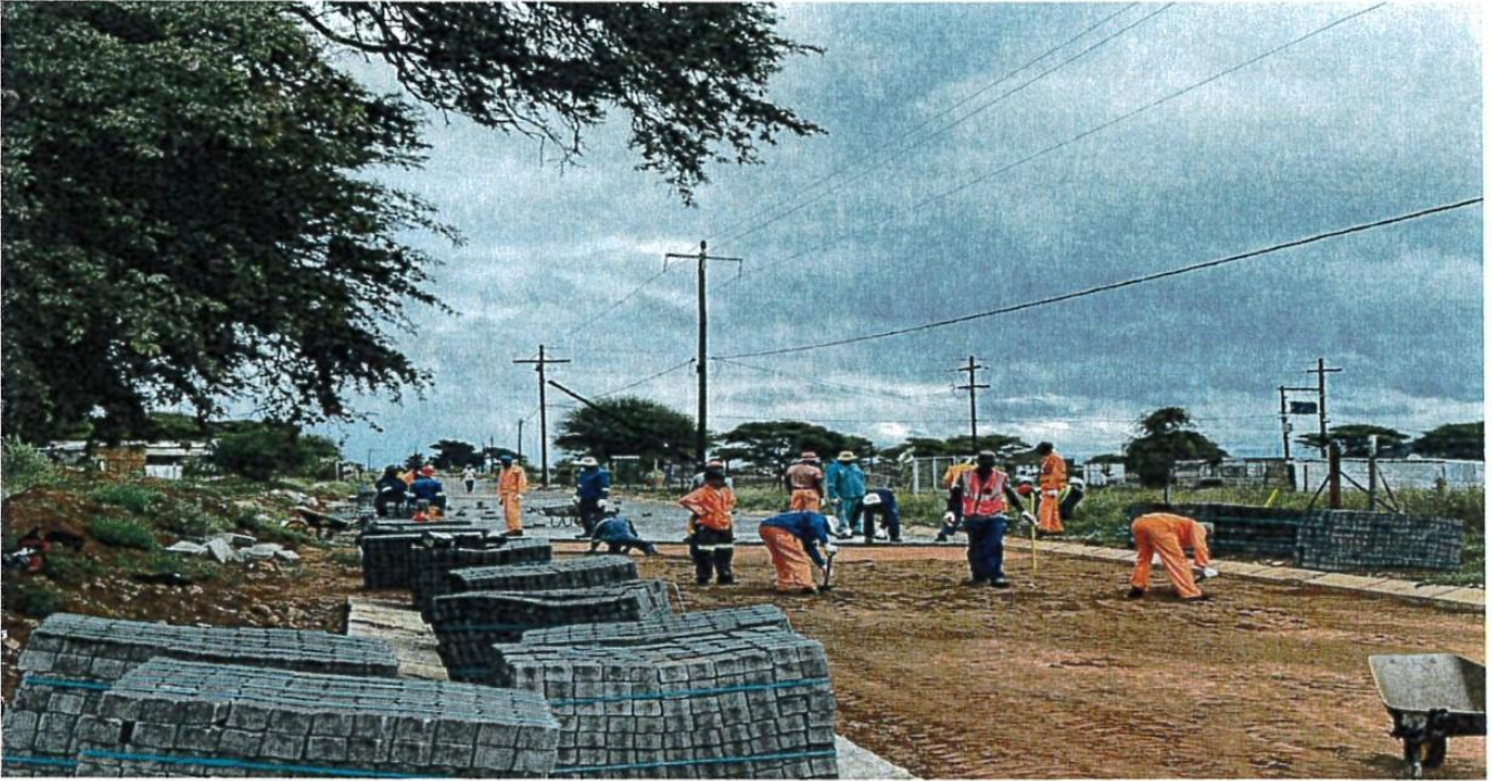
KRAALHOEK INTERNAL ROAD UNDER CONSTRUCTION AT 85%
