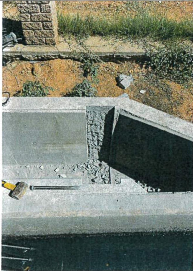
Cutting of grooves for channel gates
