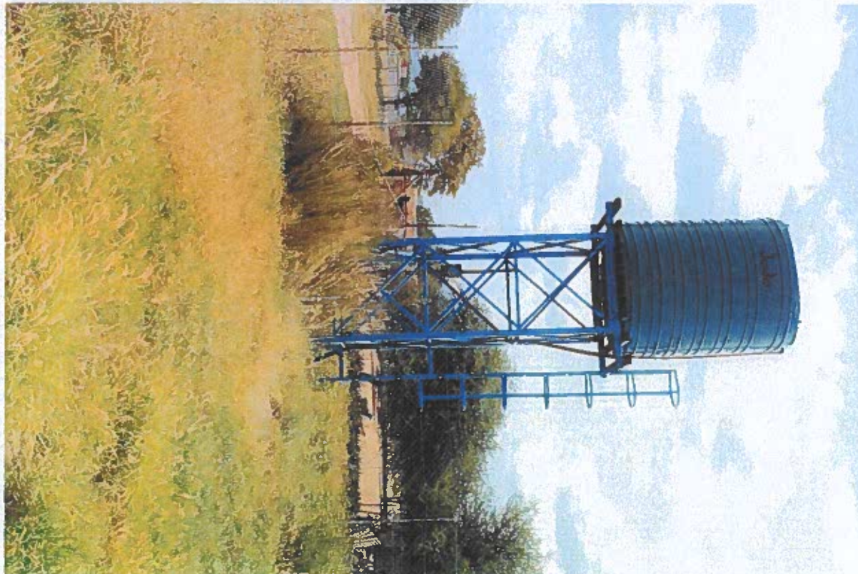
RAMOKOKA COMMUNITY HALL: WATER TANK IS LEAKING AND THE PRESSURE IS NOT ENOUGH TO FILL THE TANK AND SUPPLY THE HALL.
