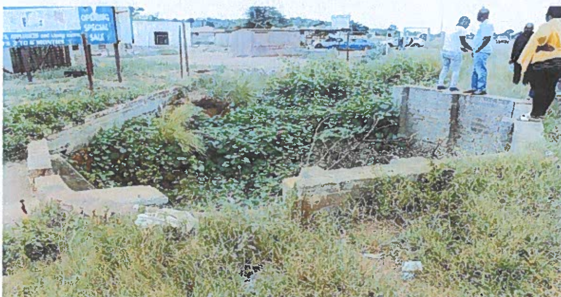
STORM WATER IN MABELE APODI: IS BLOCKED AND OTHER RESIDENTS DID BUILD THEIR HOUSES ON TOP OF IT. WATER IS NOW DIRECTED TO OTHER PEOPLES HOUSE.
