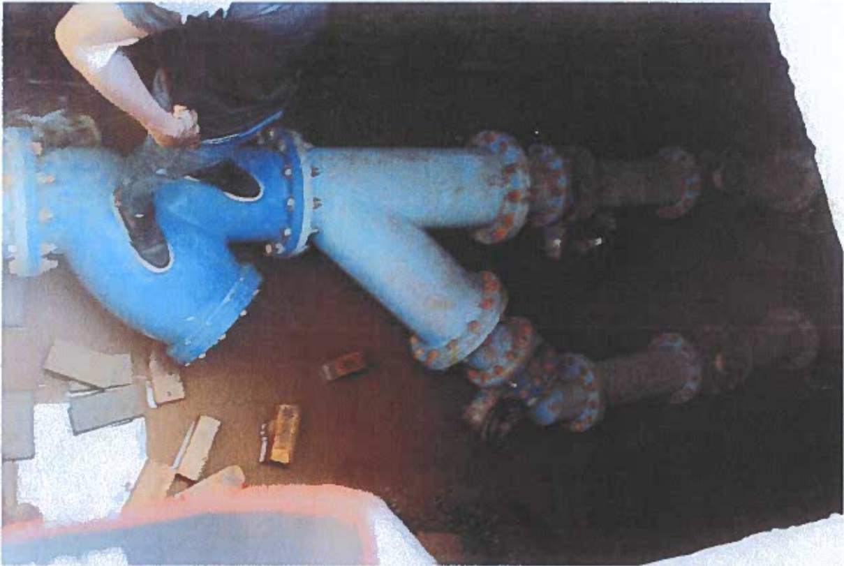
LEROME BULK WATER SUPPLY: PIPES THAT ARE INSIDE THE MANHOLE ARE LEAKING, THE BULK WATER CONNECTION HAS DRASTICALLY DROPPED BY MAGALIES FROM THE INTIAL PRESSURE LEVELS, WHICH NOW MAKES IT DIFFICULT TO SUPPLY THE SURROUNDING AREAS.
